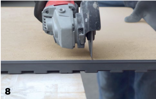
Elements can be cut with a tile cutter or angle-grinder.
