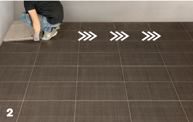
Install the first element, placing it perpendicular with the adjacent walls.
