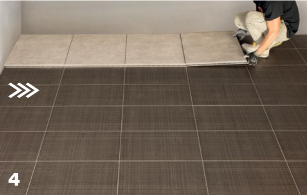
Install the first element, placing it perpendicular with the adjacent walls.
