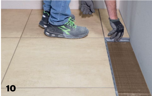
Fill any gaps between the elements and the wall with silicone.
