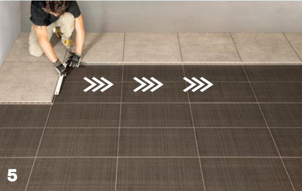
When the first row is complete, start again from the beginning, always ensuring that the elements are perpendicular.
